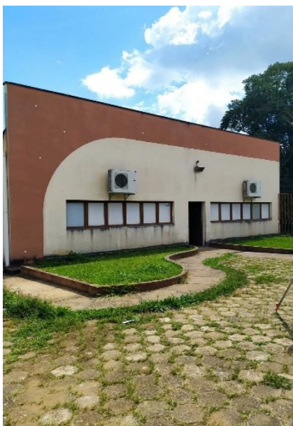
Figure 1 – LEA building facade. Source: Authors (2026).
