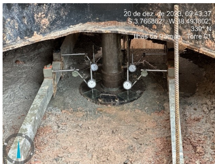
Figure 2 – Circular steel plate used in the load test. Source: Authors (2024).
