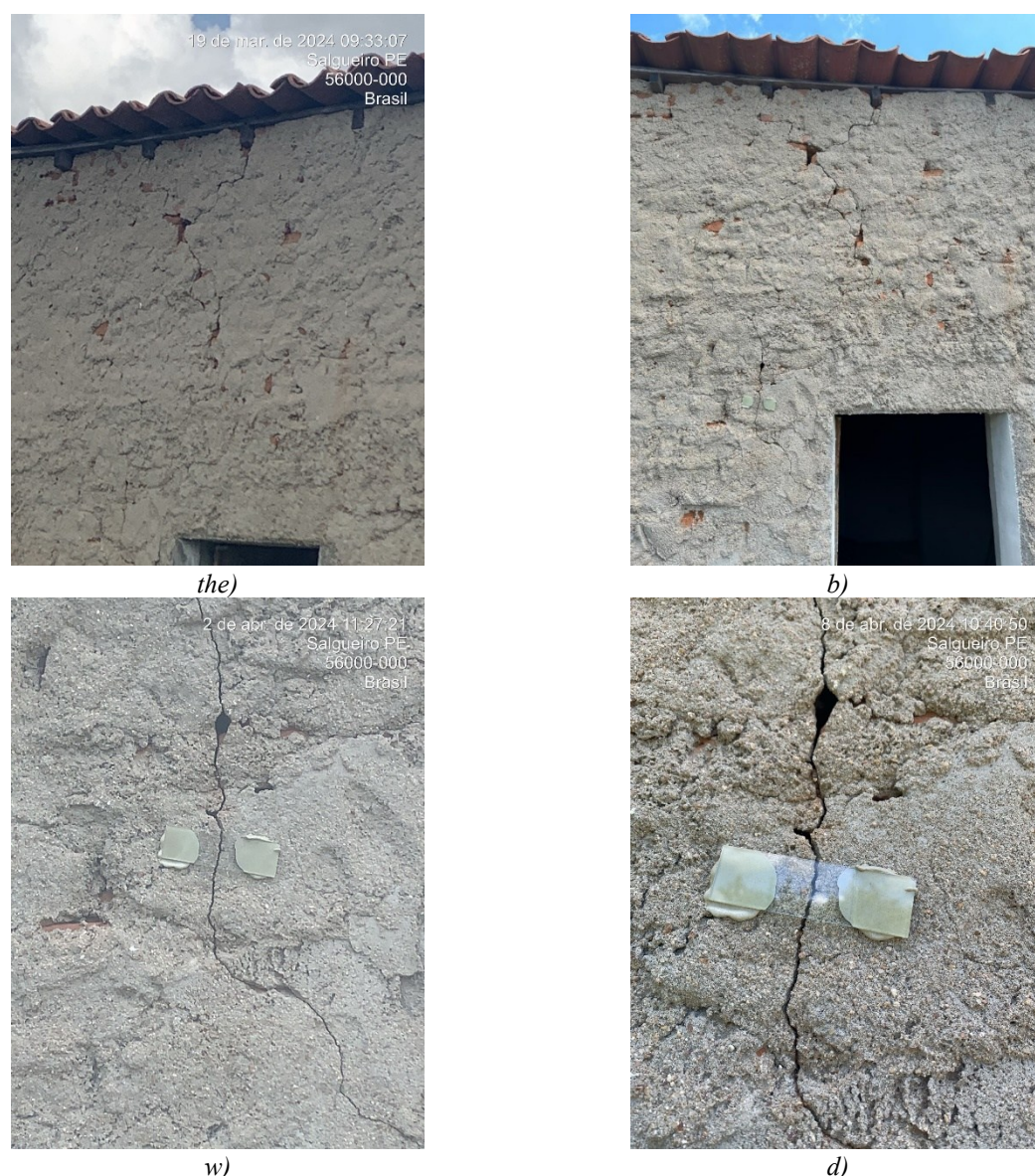
Figure 8 – Cracks in the facade cladding of the 2nd house. a) 19/03/2024. b) 25/03/2024. c) 02/04/2024. d) 08/04/2024.
