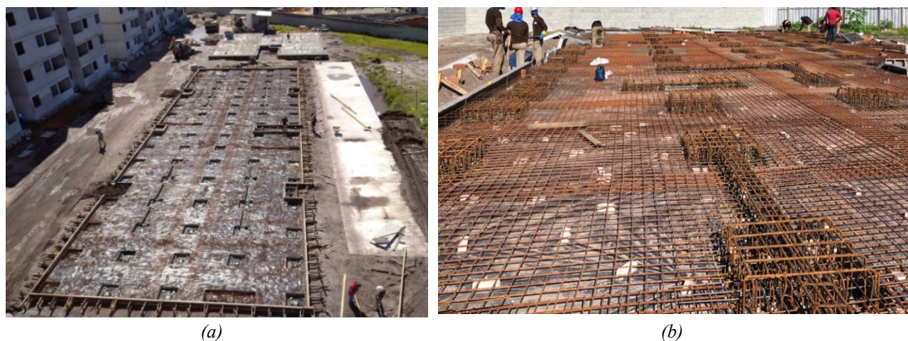
Figure 2 – (a) Location and (b) Frame of the piled raft. Source: Silva Júnior (2021).
